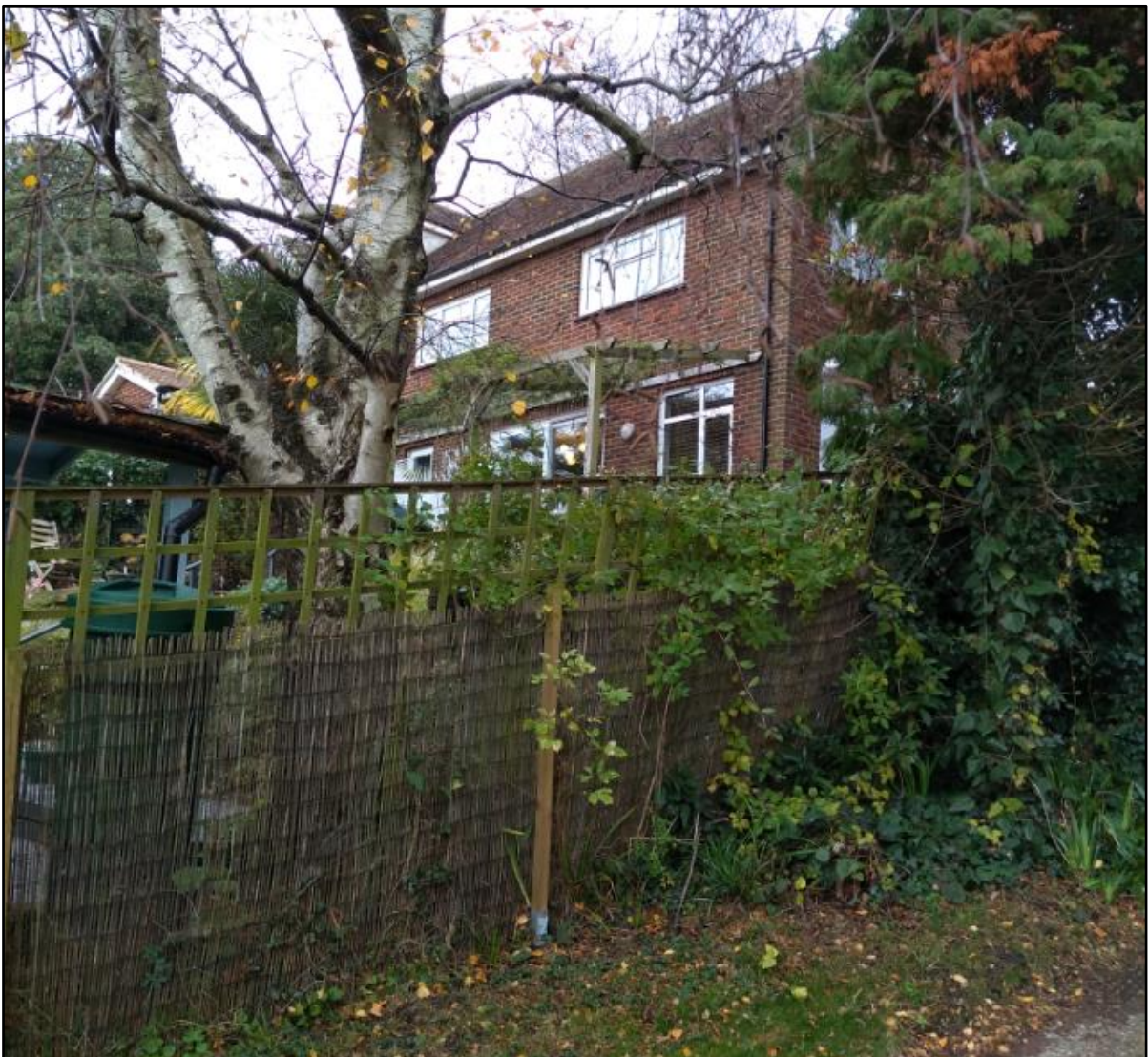
Figure 11: view from application site toward 5 North Road
